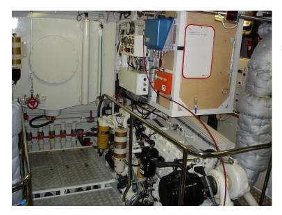
A well designed day tank, with an angled bottom and sump to encourage any dirt or water to go the lowest point, a simple drain valve with hose, clear site tube and large inspection hatch.
